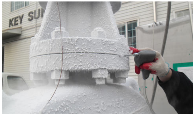
- Gasket leakage test
